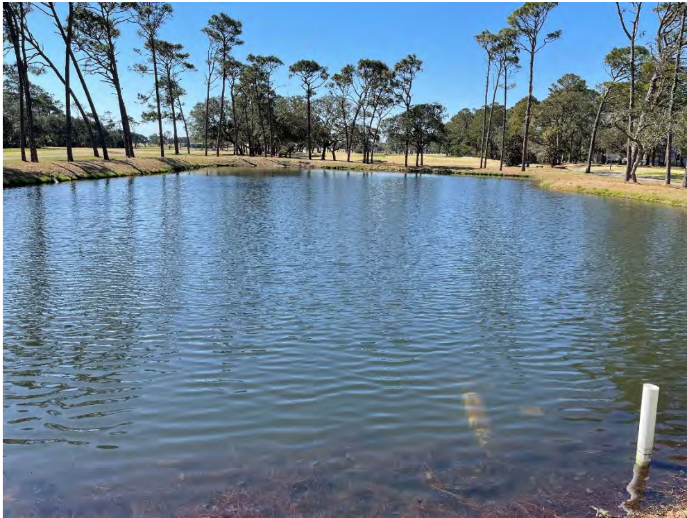
Photo 14: Ex. Infiltration Basin @ golf course for reclaimed water from SWRF.
