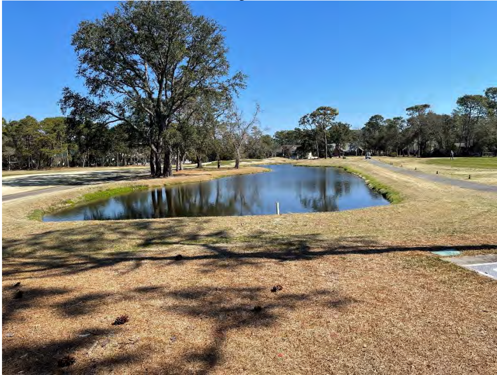
Photo 14: Ex. Infiltration Basin @ golf course for reclaimed water from SWRF.
